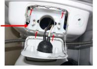
16. Clean off the old mastic from the cover and replace with non setting mastic strip or adhesive. Don't forget the cover needs to be removable!
