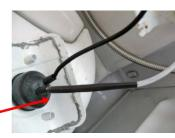
13. With a hair dryer or a heat gun gently heat the shrink wrap until it shrinks tightly over the joints. Don't overdo it and remember it maybe be hot!
