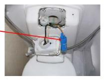
6. The connections into the switch are difficult to remove. It is better to cut the cable and join with the connectors provided.
